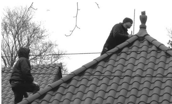
Have you noticed the terra cotta owl perched on the peak of the Children's Room roof? The owl is a copy of the 1911 Albert Entress owl that sits on the mantel in the Great Hall. It was manufactured by Ludowici Roof Tile from a model of the Entress owl cast by Bevan Ramsay. The installation of the owl marks the end of our roof restoration project, which has been documented in a scrapbook of photographs presented to the Library by John Funchion. Stop by sometime for a look.
